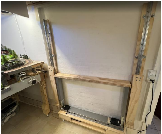
Ready for mounting the display case. The height-adjustable legs are now used to lift the display case – they are no longer attached to it.
