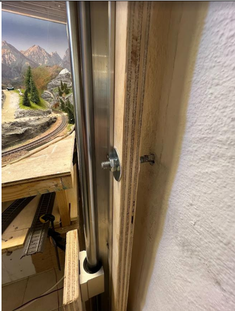
Eight M8 threaded rods per rail were installed – they were secured with Fischer injektionsmørtel
