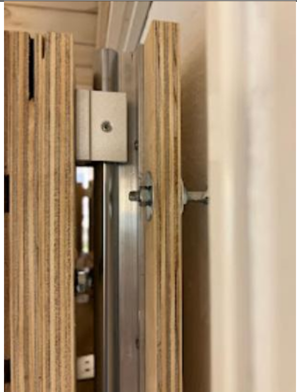
There are ball bearings in the two small carriages.
