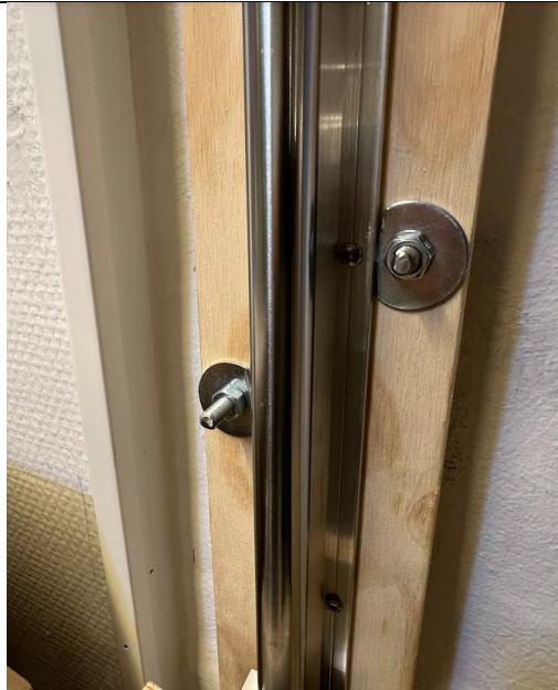
Horizontal slots were milled into the 20 mm plywood board, allowing it to be adjusted both in and out as well as sideways.
